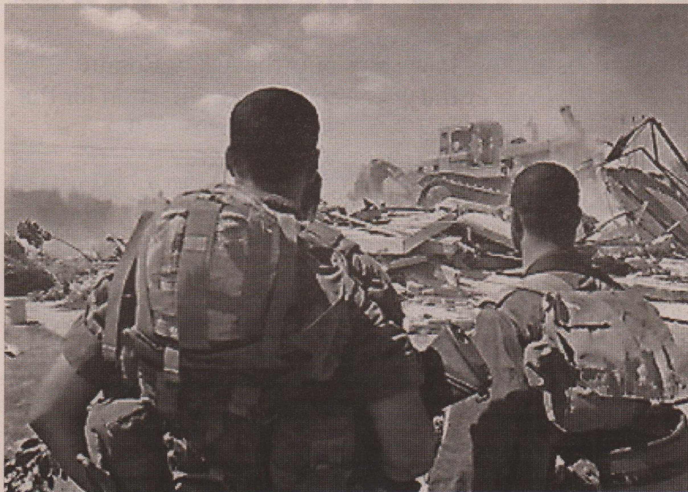
Israeli soldiers watch a bulldozer destroy a house in the former Jewish settlement of Netzer Hazani
